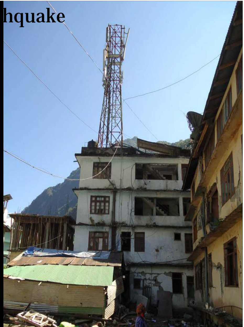
Extensive damage to buildings supporting the mobile communication towers and dish antennae
